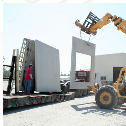
Prefab wall panels from factory, to transportation, to construction site
