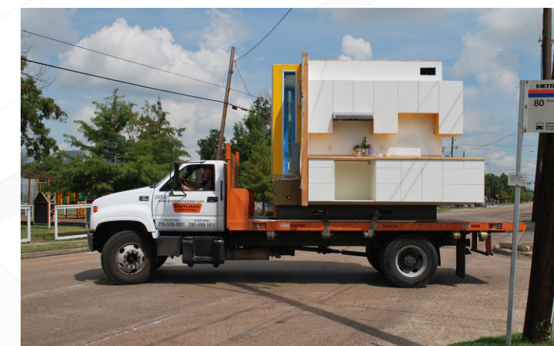
ModPod prefabricated kitchen and bathroom pod, by Rice Building Workshop
